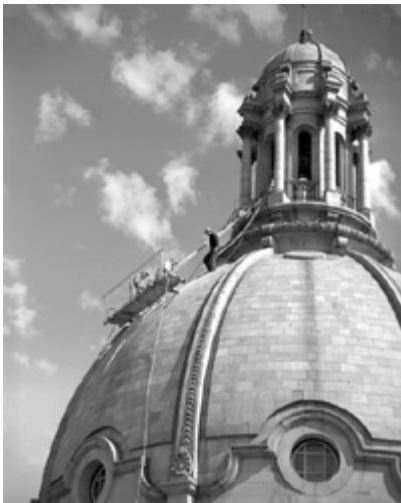
Pa40(1).9 - Repairs to the Dome of the Legislature Building, 1954, Edmonton
